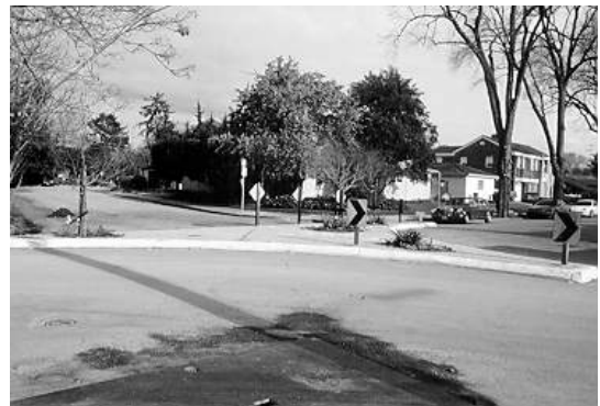
Figure 5.18. Diverter/Closure. (17th St.—San Jose, CA)
