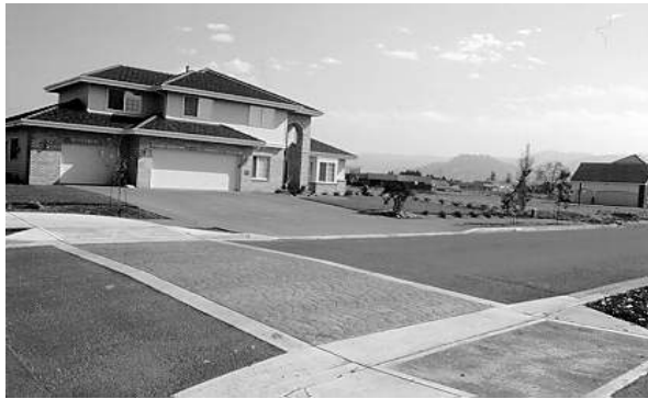
Figure 10.7. Raised Crosswalk Providing Safer Access to School. (Eugene, OR)
