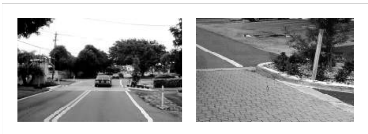
Figure 6.13. Problem Choker After Improvement. (Ft. Lauderdale, FL)
