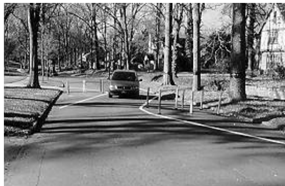
Figure 4.19. Temporary One-Lane Chicane. (Charlotte, NC)
