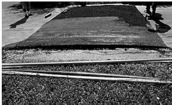
Figure 4.5. Use of Cutout to Replicate the 12-foot Parabolic Hump Profile. (Ft. Lauderdale, FL)
