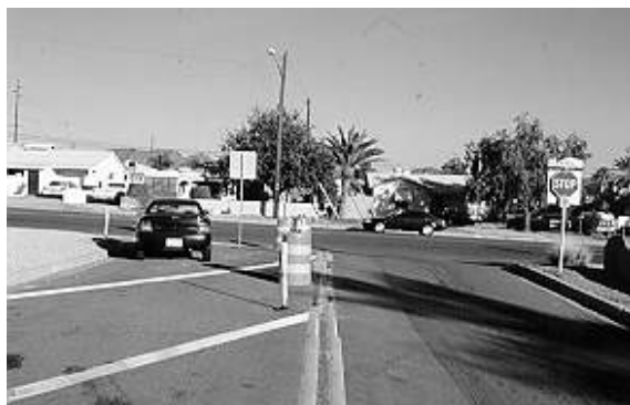
Figure 7.11. Half Closure that Invites Violations. (Phoenix, AZ)
