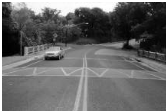
Figure 3.10. Speed Hump. (Austin, TX)
