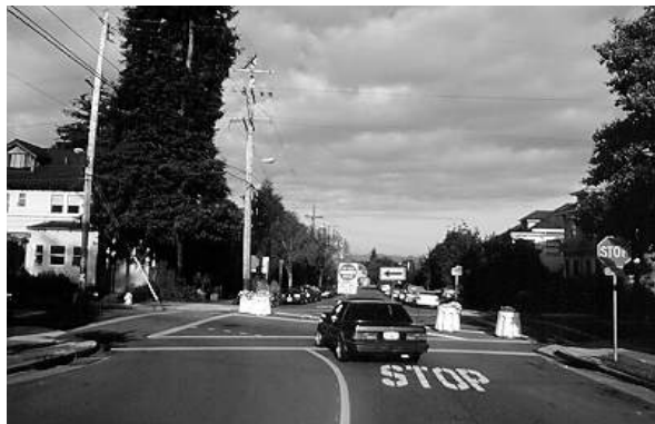
Figure 6.4. "Temporary" Diverter Challenged in Court. (Berkeley, CA)
