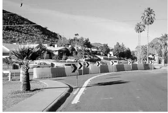
Figure 5.16. Diagonal Diverter. (6th Ave.—Phoenix, AZ)
