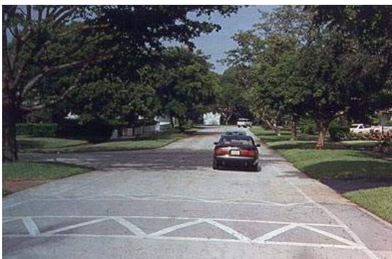
22-foot Hump. (Ft. Lauderdale, FL)
