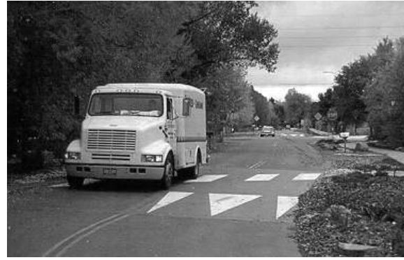
Figure 7.16. 46-foot (12 foot, 22 foot, 12 foot) Raised Crosswalk. (Boulder, CO)
