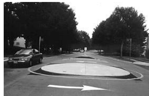
Figure 3.18. Mountable Traffic Circles. (Bellevue, WA, and Howard County, MD)
