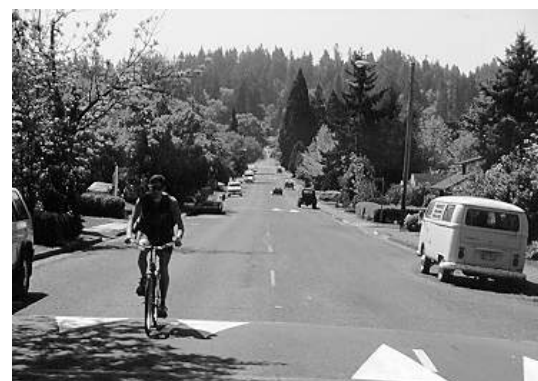
Figure 5.5. 14-foot Speed Humps. (Friendly St.—Eugene, OR)
