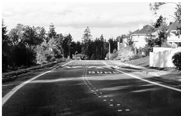
Figure 4.2. Speed Hump Enhanced by a Landscaped Choker. (Bellevue, WA)
