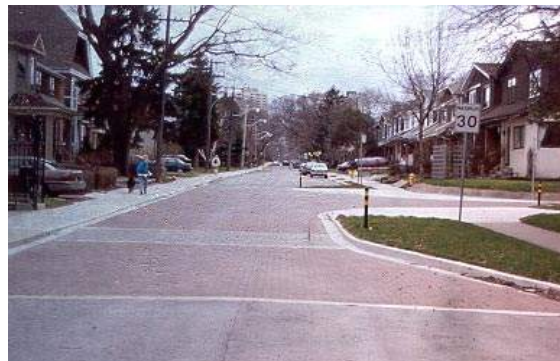
Raised Intersection with Neckdown. (Toronto, ON, Canada)
