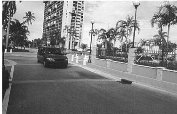
Figure 3.15. Raised Intersection. (West Palm Beach, FL)
