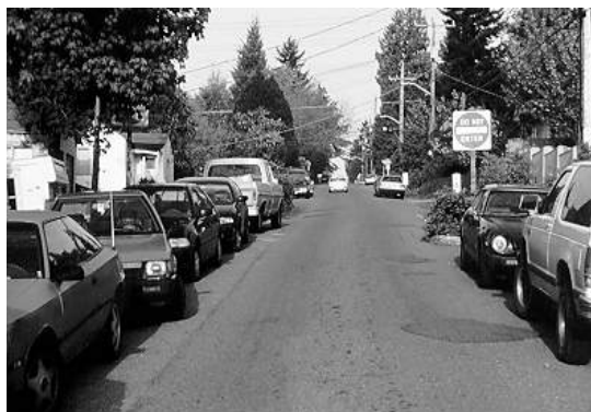
Figure 5.21. Half Closure. (NE 103rd St.—Seattle, WA)
