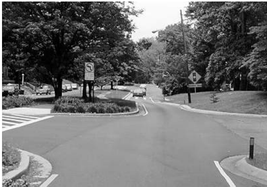
Figure 5.14. Chicanes/22-foot Speed Tables. (Huntington Pkwy.—Montgomery County, MD)
