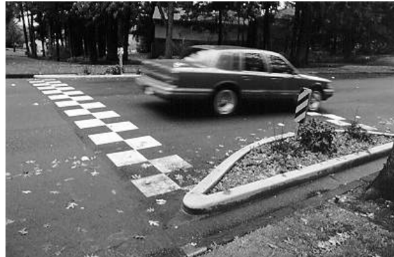
Figure 3.36. Speed Table Combined with a Choker. (Beaverton, OR)
