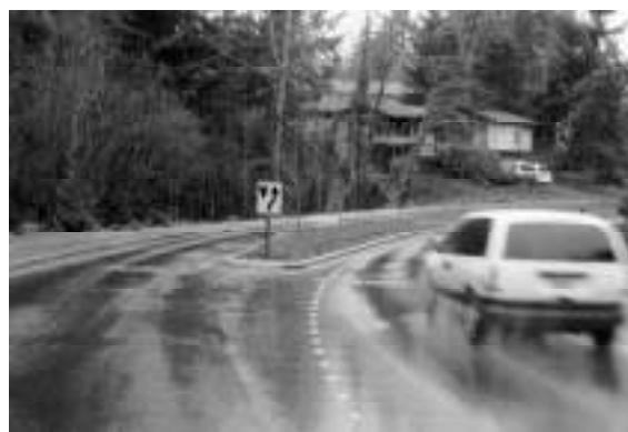
Figure 3.31. Center Island Discouraging Speeding on a Curve. (Bellevue, WA)
