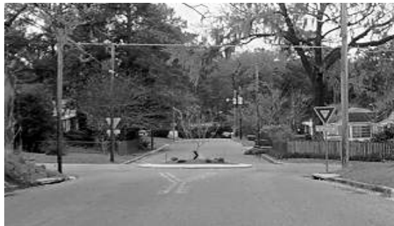
Figure 3.17. Blocking the Straight-Through Movement. (Tallahassee, FL)
