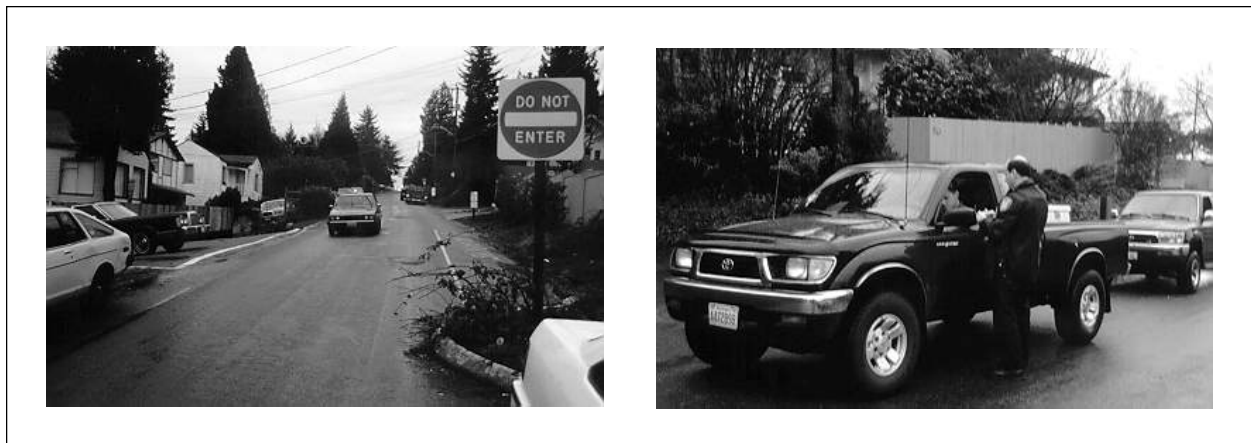
Figure 3.6. Half Closure Requiring Diligent Enforcement. (Seattle, WA)
