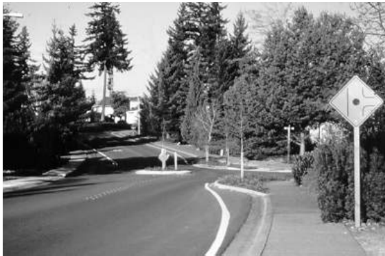
Figure 3.35. Traffic Circle Combined with Neckdowns. (Bellevue, WA)
