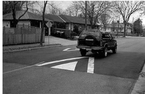
Figure 7.17. 32-foot (6 foot, 20 foot, 6 foot) Speed Table. (Minneapolis, MN)
