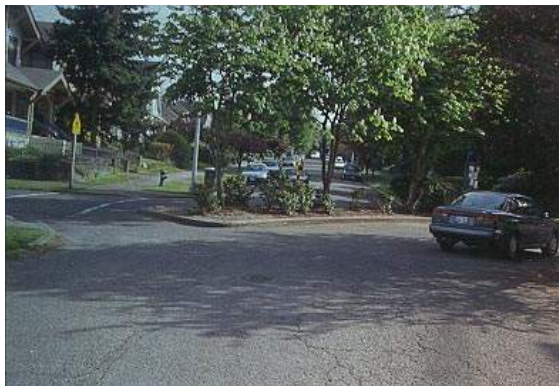
Truncated Diagonal Diverter. (Seattle, WA)
