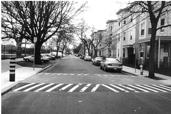
Figure 5.8. Raised Crosswalks/Raised Intersection/Chicane. (Berkshire St.—Cambridge, MA)
